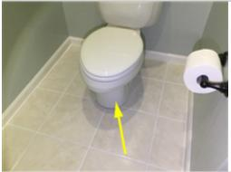
The toilet in the master bathroom rocks and is not secure to the floor. Movement of the toilet can result in leaks and damage. A licensed plumbing and general contractor should be consulted for evaluation and repair.
