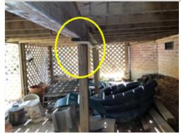
There is a post under the center of the deck that has settled and is now improperly supporting the deck structure. Improper deck construction can result in unsafe conditions and possible deck failure. A licensed general contractor should be consulted for a complete evaluation of the deck and to make necessary repairs to ensure the stability and durability of the deck.
