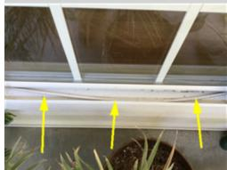
The weather-stripping for the windows on the front porch are damaged. The weather-stripping needs repair/replacement to ensure that the window is weather tight. A licensed general contractor should be consulted for evaluation and repair.
