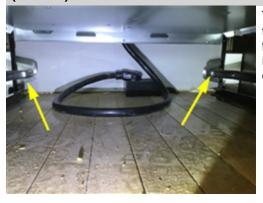
The oven moves forward when the door is opened. The oven needs to be secured or anchored with an anti-tip bracket to prevent the unit from turning over when weight is applied to the door. An appliance repair specialist or general contractor should be consulted for further evaluation and repair.
