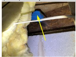
Image of the dryer duct from inside of the crawl space showing the duct taped shut and no longer in use.
