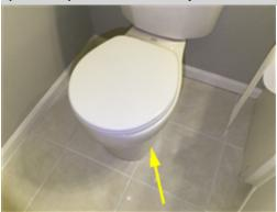
The toilet in the front center upstairs bathroom rocks and is not secure to the floor. Movement of the toilet can result in leaks and damage. A licensed plumbing and general contractor should be consulted for evaluation and repair.
