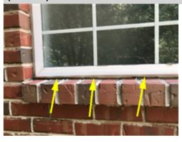
The exterior seal on the bottom of the master bathroom window is deteriorated and needs repair to stop water penetration and ensure the weather tightness of the window. The homeowner should be asked for disclosure related to the age/extent of the repair and any history of leaks. A licensed general contractor should be consulted to evaluate the extent of the damage and make necessary repairs.
