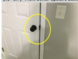
The door lock assembly in the front right upstairs bathroom is damaged/not functional. The lock could not be engaged to secure the door. The lock needs repair/replacement to ensure that the door closes securely and operates properly. A general repair specialist or licensed general contractor should be consulted for evaluation and repair.
