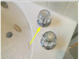
The whirlpool tub faucet is dripping/leaking. A licensed plumbing contractor should be consulted for evaluation and repair to ensure proper service.
