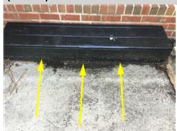
The wood step for the front porch is in direct contact with the cement walkway and there is evidence that water is directed towards the step during rain storms. A licensed general contractor should be consulted for a complete evaluation and to make necessary repairs.
