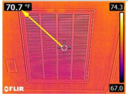
Thermal image of the temperature variance between the return/supply air for the main floor AC condensing unit. The temperature variance between the return/supply air was 12.4 degrees(F). This variance was less than typically expected, a complete evaluation by an HVAC contractor is needed.
