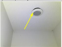
The light fixture in the pantry off the kitchen is damaged. Damaged fixtures could result in improper operation and electrical hazards. A licensed electrical contractor should be consulted for further evaluation and repair.
