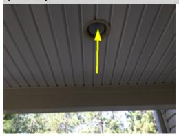
One of the front porch lights was not functional when tested. This could indicate a defective bulb or other more serious problem such as faulty wiring or a defective fixture. A licensed electrical contractor should be consulted for further evaluation and repair.
