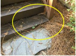
The bottom step to the rear wood deck has settled, is in direct contact with the ground and is decayed/deteriorating. A licensed general contractor should be consulted to review the steps and repair as needed to ensure safe access and egress.
