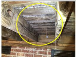
The underside of the wood deck was found to be weathered. A licensed general contractor should be consulted for a complete evaluation of the deck and to make necessary repairs to ensure the stability and durability of the deck.
