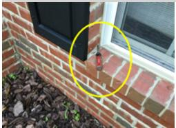
There is a gap at the bottom left side of the garage window between the window and the brick veneer. The gap could indicate a problem with the window installation or movement of the brick veneer. A licensed general contractor should be consulted for a complete evaluation of this and other windows to determine the significance of the concern and outline necessary repairs.
