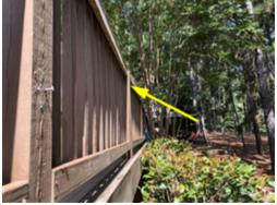
The railings on the back of the deck are loose in a couple of areas and present a safety/fall hazard. A licensed general contractor should be consulted for evaluation of the deck handrail system and to make necessary repairs.
