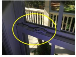
The window on the left hand side of the dining room needs repair to ensure proper operation. The window did not properly latch, lock, open. All windows should be evaluated as repairs are made. A licensed general contractor should be consulted to review the installation and repair as needed to ensure safe and secure operation.
