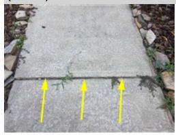
The sidewalk is raised, cracked, uneven along the walking surface resulting in a trip hazard. A licensed general contractor should be consulted for further evaluation and repair.
