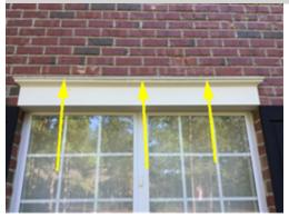
Wood decay was noted above the large garage window. Decay in the windows can result in leaking and water penetration and should be repaired as soon as possible. All windows should be evaluated for damage and or decay behind the trim as repairs are made. A licensed general contractor should be consulted to evaluate the extent of the damage and to make necessary repairs.
