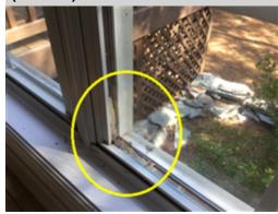
At least two of the windows in the breakfast nook area have started to decay inside the frame area and there is a lot of debris present at the bottom inside of the panes. All windows should be evaluated as repairs are made. A licensed general contractor should be consulted.
