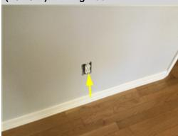
There are two receptacles in the dining room that do not have a protective cover plate. This could result in increased shock and fire hazards. A licensed electrical contractor should be consulted to make necessary repairs to ensure safe and proper operation and installation.
