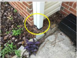
The gutter downspouts around the home are piped underground, however the exits were not located or verified. Direct drainage to the foundation and cladding from the gutter system can result in water penetration into the foundation area and foundation deterioration. A licensed general contractor should be consulted for a complete evaluation to locate and verify the downspout extension and to make necessary repairs.
