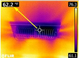
Thermal image of the temperature variance between the return/supply air for the main floor AC condensing unit. The temperature variance between the return/supply air was 11.7 degrees(F). This variance was less than typically expected, a complete evaluation by an HVAC contractor is needed.
