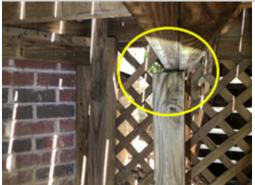
There is a post under the main part of the deck near the staircase that is kicked out and is no longer vertical. Improper deck construction can result in unsafe conditions and possible deck failure. A licensed general contractor should be consulted for a complete evaluation of the deck and to make necessary repairs to ensure the stability and durability of the deck.
