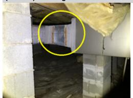
Parts of the metal housing for the Heating Unit in the crawl space has visible areas of rust that is likely due to long term presence of moisture. An HVAC contractor should be consulted for a complete evaluation and to make necessary repairs to ensure safe, reliable, and proper operation of the HVAC system.
