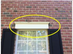
Wood decay was noted above the small garage window. Decay in the windows can result in leaking and water penetration and should be repaired as soon as possible. All windows should be evaluated for damage and or decay behind the trim as repairs are made. A licensed general contractor should be consulted to evaluate the extent of the damage and to make necessary repairs.
