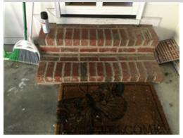
The bottom step at the entrance of the home from the garage has a noticeable variance in the height. This configuration could result in the trip or fall hazard as someone enters or leaves the home. A licensed general contractor should be consulted to review the steps and repair as needed to ensure safe access and egress.
