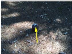
The main waste line is exposed above grade in the back yard of the home. The waste line should be below grade to protect it from damage and extreme temperatures. A licensed plumbing contractor should be consulted for a complete evaluation and to make necessary repairs.
