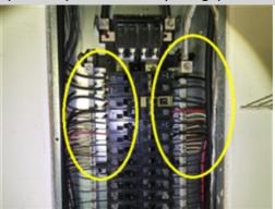
There are a number of breakers on the left/right side of the electrical panel has a conductor and ground wire attached to the power screw. This condition presents a safety hazard that could result in interrupted service, property damage, and serious personal injury. A licensed electrical contractor should be consulted for further evaluation to verify the breaker rating and to make necessary repairs.
