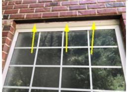
The exterior seal on the top of the master bathroom window is deteriorated and needs repair to stop water penetration and ensure the weather tightness of the window. The homeowner should be asked for disclosure related to the age/extent of the repair and any history of leaks. A licensed general contractor should be consulted to evaluate the extent of the damage and make necessary repairs.
