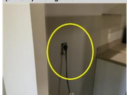
The receptacle behind the fridge does not have a protective cover plate. This could result in increased shock and fire hazards. A licensed electrical contractor should be consulted to make necessary repairs to ensure safe and proper operation and installation.
