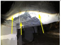
The insulation for the duct system attached to the main Heat Pump unit in the crawl space was noted to be spongy and wet. The source of the moisture and any related concerns need to be addressed to ensure proper air flow and prevent contamination of the air supply. An HVAC contractor should be consulted for a complete evaluation and replacement of all damaged duct components to ensure reliable and proper operation of the HVAC system.
