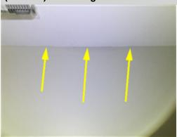
Stains on the ceiling in the large front right upstairs bedroom indicate a history of a leak. At the time of the inspection it was not possible to determine if the condition was due to an active or past occurrence. Further investigation by a repair specialist and owner disclosure is recommended. Refer to the Attic section of the report.
