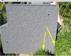
There are a number of tree limbs either in contact with the home/roof or starting to grow over the roof. Keeping trees trimmed and spaced away from the roof, wall cladding and foundation provides air circulation. It is recommended that an arborist be consulted to evaluate and/or trim the trees.
