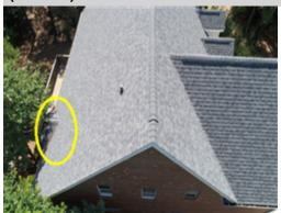
A couple of the valleys on the rear part of the roof covering are covered with a heavy build-up of leaves/pine needles/debris. This limited the inspection of the roof surface. Debris on the roof surface can trap moisture allowing water and debris to travel under the shingle tabs resulting in material failure and leaks. A roofing contractor should be consulted to remove the debris and inspect the shingles/adjacent component for evidence of damage and make necessary repairs.
