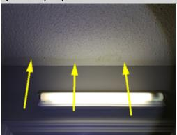
Stains on the ceiling in a bedroom closet upstairs indicate a history of a leak. At the time of the inspection it was not possible to determine if the condition was due to an active or past occurrence. Further investigation by a repair specialist and owner disclosure is recommended. Refer to the Attic section of the report.
