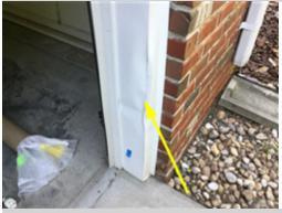
The garage door needs adjustment and repair. The right side panel is bent/damaged. A garage door installation company or a licensed general contractor should be consulted for evaluation and repair to ensure that the door operates safely and properly.
