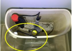
The toilet flush valve is not operating properly. This could result in improper functioning, flooding and waste of water. A licensed plumbing contractor should be consulted for evaluation and repair.
