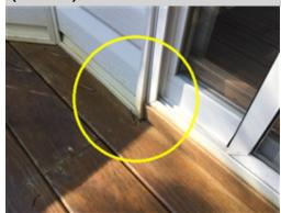
The vinyl siding at the bottom left side of the sliding patio door is damaged and pulling away from the structure. A licensed general contractor should be consulted for complete evaluation to locate and repair all areas of damage.
