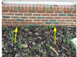
The grading around the foundation at the front of the home has become too high and is partially covering the weep holes. Years of bedding and wood chips has brought the bedding level to or above the slab interior floor level. Incorrect clearance can result in water penetration, drainage, and conditions inducive of insects and decay. A licensed general contractor should be consulted to evaluate and correct the grading as needed for proper clearance and drainage.
