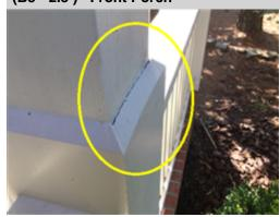
Some of the front porch columns are weathered and starting to split. Repair and painting is needed to prevent further damage and decay. A general repair person should be consulted.
