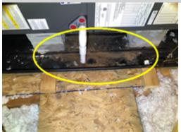
The auxiliary drain pan underneath the Heat Pump Unit in the attic has evidence of rust. This condition indicates a history of improper drainage of the system condensate water. Improper drainage of the condensate water can result in system and property damage. An HVAC contractor should be consulted for a complete evaluation and to make necessary repairs to ensure safe, reliable, and proper operation of the HVAC system.
