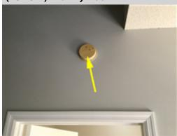
This home has a limited number of smoke detectors as compared to current standards and the inspector could not confirm the presence of Carbon Monoxide detectors. Currently is it recommended that a smoke/carbon dioxide detector be installed at each floor level in the home and in each sleeping room. Correction is recommended.
