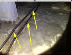
The AC refrigerant line sets that connects the outside compressor units to the interior air handler are in direct contact with the ground of the crawl space. An HVAC contractor should be consulted for a complete evaluation and repair of the system to ensure reliable and proper operation of the HVAC system.
