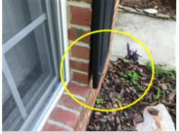
The shutter to the right of the large garage window is not secure to the exterior of the home. A general contractor should be consulted to ensure this and other shutter's are properly secured to the home.
