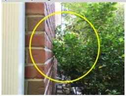
The vegetation around the perimeter of the home is over grown and blocks the air circulation around the home. The growth also limited the inspection access. A landscaping company should be consulted to correct the over growth and the inspection should be completed prior to purchase.
