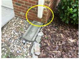
The gutter downspout to the right of the garage is not extended or piped to direct roof drainage away from the foundation. Direct drainage to the foundation and cladding from the gutter system can result in water penetration into the foundation area and foundation deterioration. A licensed general contractor should be consulted for a complete evaluation and to make necessary repairs.
