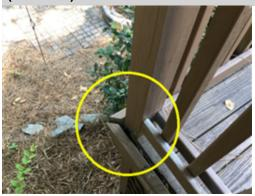
The facia boards on the rear deck near the stair case are separating. A licensed general contractor should be consulted for a complete evaluation and to make necessary repairs to ensure the boards are secure to prevent cupping and possible trip hazards.
