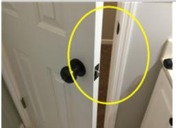
The door lock assembly in the upstairs hallway bathroom is damaged/not functional. The lock could not be engaged to secure the door. The lock needs repair/replacement to ensure that the door closes securely and operates properly. A general repair specialist or licensed general contractor should be consulted for evaluation and repair.
