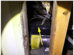
The whirlpool pump motor has not been bonded as required for homes with copper or metal plumbing. A licensed electrical contractor should be consulted for evaluation and repair to ensure safe and proper operation.
