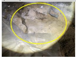
The soil on the left side of the crawl space is severely eroded and has left a portion of the crawl space foundation unsupported. An engineer should be consulted to determine the significance of the concerns and for a full evaluation of the foundation to outline necessary repairs.
