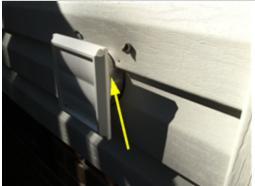
There is an old dryer duct at the rear of the home near the deck staircase that is not properly secured to the exterior cladding of the home. Upon further investigation the inspector confirmed that this duct has been taped over inside the crawl space and another duct is now running to the left side of the home near the garage door. A licensed general contractor or general repair specialist should be consulted for further evaluation and to make necessary repairs.
