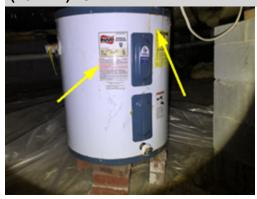
The water heater installed in the crawl space is in poor condition and at the time of the inspection it appeared that the unit was no longer level. A licensed plumbing contractor should be consulted to evaluate the condition of the unit and correct the installation to prevent damage.
