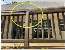
The railing on the back, center of the deck are damaged. A licensed general contractor should be consulted for evaluation of the deck handrail system and to make necessary repairs.
