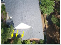
The gutters around the home have excess debris, pine needles and leaves. Direct drainage to the foundation and cladding from the gutter system can result in water penetration into the foundation area and foundation deterioration. A licensed general contractor should be consulted for a complete evaluation and to make necessary repairs.
