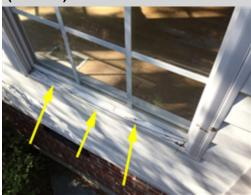
The weather-stripping for the windows on the back deck are damaged. The weather-stripping needs repair/replacement to ensure that the window is weather tight. A licensed general contractor should be consulted for evaluation and repair.
