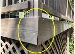
The facia boards on the back right area of the rear deck are separating. A licensed general contractor should be consulted for a complete evaluation and to make necessary repairs to ensure the boards are secure to prevent cupping and possible trip hazards.
