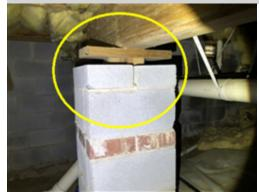
The pier located on the center right side of the crawl space is not plumb or vertical. This could indicate that the pier is leaning, the pier footing has failed, or that the pier has moved. A licensed general contractor should be consulted for further evaluation and to make necessary repairs.
