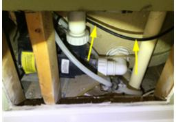
The whirlpool could not be verified to be protected by a GFCI circuit. A GFCI is needed to ensure safe and functional operation of the tub. A licensed electrical contractor should be consulted for evaluation and repair.
