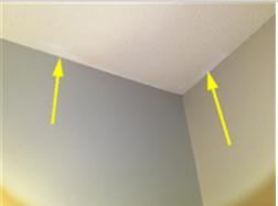
Evidence suggests that the ceiling in the powder room has been repaired/painted. The owner should be asked for disclosure related to the extent of any related repairs, leaks or problems and the reason the ceiling was painted. New paint can limit the inspection as all history of defects or concerns are not visible.
