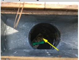
Many of the main floor ducts are filled with garbage and debris. The debris reduces the air flow and contaminates the air supply. An HVAC contractor should be consulted for a complete evaluation and replacement of all damaged duct components to ensure reliable and proper operation of the HVAC system.
