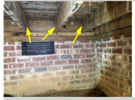
The floor joists for the deck are supported or attached to the home by toe nail connections only. Nails can corrode and fail leaving the floor system unsupported. Improper deck construction can result in unsafe conditions and possible deck failure. A licensed general contractor should be consulted for a complete evaluation of the deck and to make necessary repairs to ensure the stability and durability of the deck.
