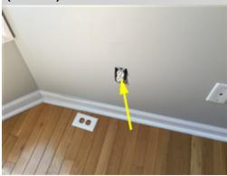
A receptacle in the master bedroom whose protective plate is not installed. This could result in increased shock and fire hazards. A licensed electrical contractor should be consulted to make necessary repairs to ensure safe and proper operation and installation.
