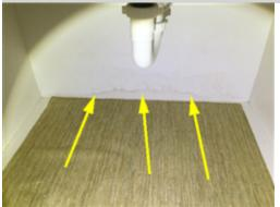
There is evidence of a leak in the cabinet underneath the sink in the upstairs hallway bathroom. The inspector could not determine whether this was an active or current leak. The owner should be asked for information regarding a leak in this area of the home and if required, a plumbing contractor should be consulted to assess this area of the home and recommend repairs.
