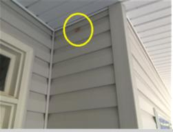
There is evidence of wasps on the exterior siding to the right of the front door. A licensed pest contractor should be consulted for a complete evaluation of the exterior siding to remove this and any other pests on the exterior of the home.
