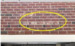
It appears that a small area of bricks above the garage door have been repaired/new mortar applied. Deteriorated mortar could indicate defects related to age, water penetration, or improper installation. Homeowner disclosure and a masonry contractor should be consulted for further evaluation of the brick veneer and to repair all loose, soft, missing mortar.
