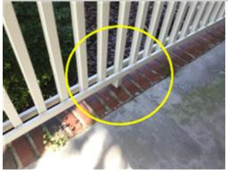
The railings for the front porch are loose and in need of repair or replacement to ensure safe and functional use of the front porch. A licensed general contractor should be consulted for a complete evaluation and to make necessary repairs.
