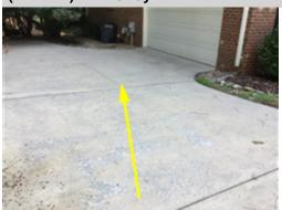
The driveway is sloped to encourage storm drainage to flow toward the home. Efflorescence in the front left area of the crawl space indicate that lot drainage from the driveway area is entering the crawl space area. Drainage into the crawl space can result in damage to the home. A licensed general contractor should be consulted for further evaluation and repair.
