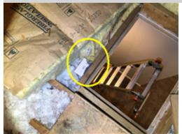
The plate for the light switch used to turn on the attic light is broken. A licensed electrical contractor should be consulted for a complete evaluation to determine the significance of this concern and make necessary repairs to correct defects and prevent safety hazards.
