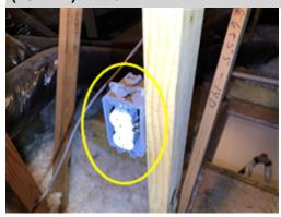
Electrical connections have been made in the attic area without being properly protected in a covered junction box. The open junction leaves electrical conductors exposed and in a hazardous condition. Electrical concerns should be considered fire and safety issues and repaired as soon as possible. The electrical systems and components in the attic are in need of a complete evaluation and repair by a licensed electrical contractor.
