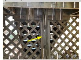
There is a post under the deck attached to the staircase that is no longer vertical. Improper deck construction can result in unsafe conditions and possible deck failure. A licensed general contractor should be consulted for a complete evaluation of the deck and to make necessary repairs to ensure the stability and durability of the deck.
