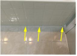
The grout/caulking where the tile meets the whirlpool tub needs repair. New caulking has been installed below the entrance to the shower stall. The purpose of the grout/caulk is to fill the space between the tiles and to protect the bond between the tile and the mortar base. A tile installation/repair company should be consulted to evaluate the tile system to determine the significance of the concern and make necessary repairs.
