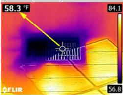
Thermal image of the temperature variance between the return/supply air for the main floor AC condensing unit. The temperature variance between the return/supply air was 12.4 degrees(F). This variance was less than typically expected, a complete evaluation by an HVAC contractor is needed.
