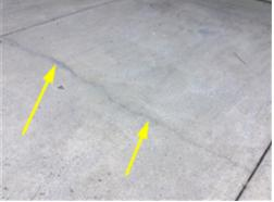
The driveway is cracked. The crack may provide a path for water penetration under the slab. A licensed general contractor should be consulted for further evaluation and repair.
