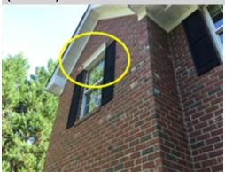
Wood decay was noted above the front left bedroom window. Decay in the windows can result in leaking and water penetration and should be repaired as soon as possible. All windows should be evaluated for damage and or decay behind the trim as repairs are made. A licensed general contractor should be consulted to evaluate the extent of the damage and to make necessary repairs.
