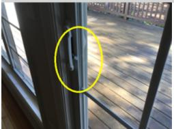
The locking mechanism for the sliding patio door is damaged and does not operate as intended. The door needs repair/replacement to ensure that the it closes securely and operates properly. A general repair specialist or licensed general contractor should be consulted for evaluation and repair.
