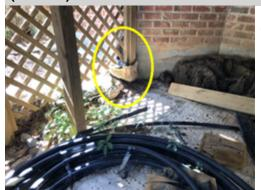
Some of the wood deck posts are supported by poured cement footings. The poured footing on the right side of the deck nearest the home is no longer in contact with the ground and therefore not providing the necessary and required support. Incorrect post footings could allow the structure to move or fail. A licensed general contractor should be consulted for a complete evaluation of the deck and to make necessary repairs to ensure the stability and durability of the deck.
