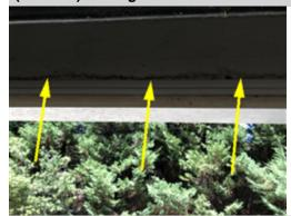
Stains above the garage door on the inside indicate that water has entered the garage area adjacent to or around the metal lintel. A licensed general contractor should be consulted to determine the significance of this concern and to make necessary repairs.
