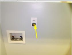
The home was built before GFCI circuits were required to protect all electrical receptacles located within six feet of water. GFCI circuits add an important safety feature to electrical systems. The buyer should consider upgrading the electrical system to include GFCI protection.
