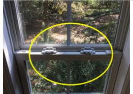
The single window to the right of the breakfast nook looking to the back yard is damaged and doesn't open/close properly. This could indicate a problem with the window and or trim installation. A licensed general contractor should be consulted to determine the cause of the separation and repair as needed.
