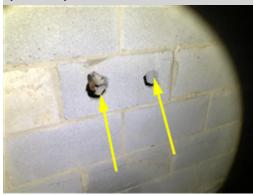
There are two holes in a cinder block brick on the back wall foundation in the crawl space. The purpose of these holes could not be determined at the time of the inspection. It doesn't appear that these holes have impacted the structural fitness of the foundation. If the buyer is concerned about these holes, an engineer should be consulted.
