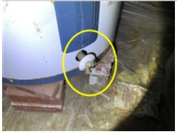
The water heater is equipped with a drain valve in the lower region of the tank. Water heaters need to be drained for maintenance, repair, and replacement. The valve for this unit was noted to be damaged and in need of repair. A licensed plumbing contractor should be consulted to evaluate the system and repair/replace as needed to ensure safe and reliable hot water supply.
