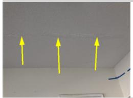
There is evidence of damage/repairs on the ceiling of the garage that may indicate a history of a leak. At the time of the inspection it was not possible to determine if the condition was due to an active or past occurrence. Further investigation by a repair specialist and owner disclosure is recommended.
