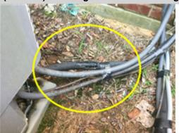
The large line of the AC refrigerant line set that connects the Carrier outside compressor unit to the interior air handler is required to be insulated to reduce condensation and associated water damage. The AC line insulation is missing/damaged near the connection to the unit. An HVAC contractor should be consulted for a complete evaluation and repair of the system to ensure reliable and proper operation of the HVAC system.
