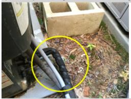
The large line of the AC refrigerant line set that connects the Goodman outside compressor unit to the interior air handler is required to be insulated to reduce condensation and associated water damage. The AC line insulation is missing/damaged near the connection to the unit. An HVAC contractor should be consulted for a complete evaluation and repair of the system to ensure reliable and proper operation of the HVAC system.
