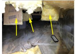
The insulation is/has been wet due to leaks or elevated area moisture levels and is missing, hanging or has fallen to the floor of the crawl space. Typically insulation must be replaced if it has been wet because it does not retain fire protective coatings. The insulation needs to be replaced and the adjacent areas inspected for damage. A licensed general contractor should be consulted for repair/replacement.
