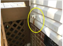
During the inspection, there is a rust stain on the exterior of the home where the drain exit for the AC condensate exits the crawl space. An HVAC contractor should be consulted for a complete evaluation and repair of the system to ensure reliable and proper operation of the HVAC system.
