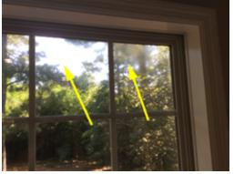
At least two of the windows in the breakfast nook have a cloudy or hazed appearance. The cloudy appearance indicates that the gas seal between the double glass panes has been jeopardized reducing the energy rating of the windows. The severity of the hazing varies with season and time of the day; therefore, all damaged windows may not have been visible at the time of the inspection. All windows should be evaluated as repairs are made. A licensed general contractor should be consulted.
