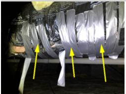
The insulation cover for duct branches near the front of the crawl space are deteriorated, damaged and have been repaired with duct tape. The cover protects the duct structure and holds the insulation in place. An HVAC contractor should be consulted for a complete evaluation and replacement of all damaged duct components to ensure reliable and proper operation of the HVAC system.
