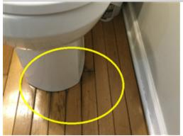
The wood flooring around the toilet in the main floor powder room shows evidence of a previous water leak. A licensed general contractor should be consulted for an invasive investigation to determine the source of the water penetration and the extent of the decay to prevent further damage and undesirable conditions.
