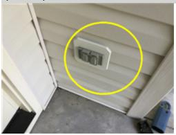
The receptacle on the front porch to the right of the front door is loose. Loose receptacles could result in electrical shock hazard or property damage. A licensed electrical contractor should be consulted for a complete evaluation to determine the significance of this concern and make necessary repairs to correct defects and prevent safety hazards.
