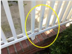
Some of the styles on the front porch columns are weathered and in need of paint to avoid decay and further damage. Repair and painting is needed to prevent further damage and decay. A general repair person should be consulted.
