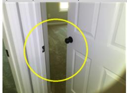
The door lock assembly in the front left upstairs bedroom is damaged/not functional. The lock could not be engaged to secure the door. The lock needs repair/replacement to ensure that the door closes securely and operates properly. A general repair specialist or licensed general contractor should be consulted for evaluation and repair.
